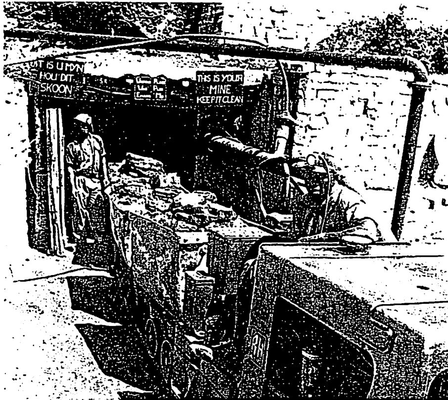
The broken asbestos-bearing rock – ten parts of asbestos to a hundred parts of rock – is brought to the surface by diesel train
