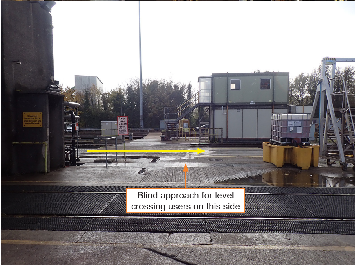
Figure 10: The blind corner at the end of the main shed building.
