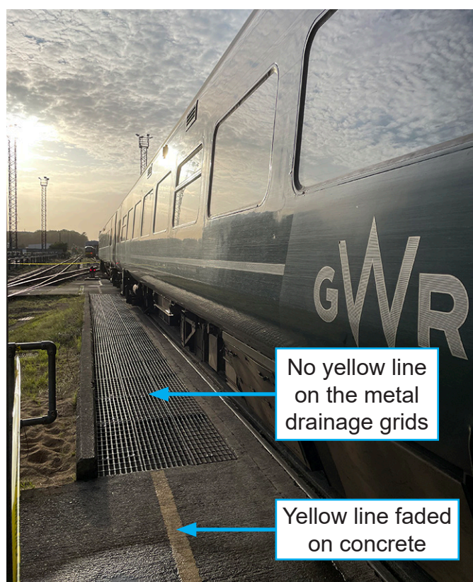
Figure 15: The faded yellow lines along the walkway.
