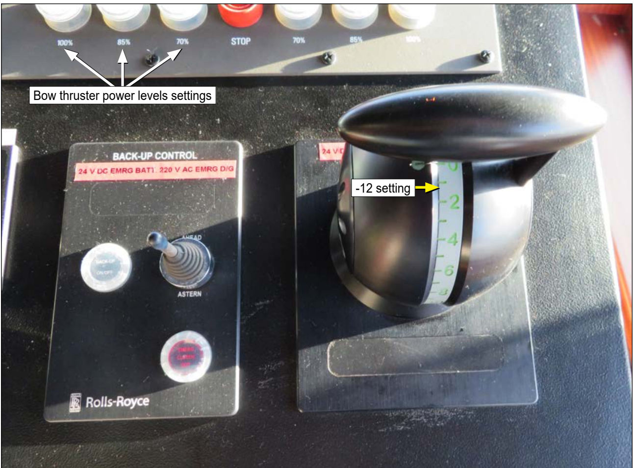
Figure 10: Propulsion control unit
