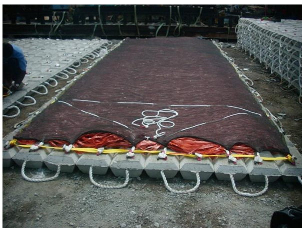
Figure 2.4.18: Typical concrete and concrete froned mattresses (6m x 3m x 0.15m)
