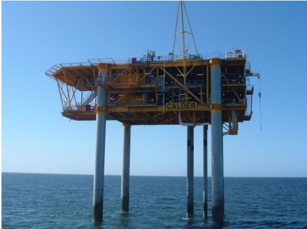
Figure 2.1.4: Photograph of the Calder platform (south face)
