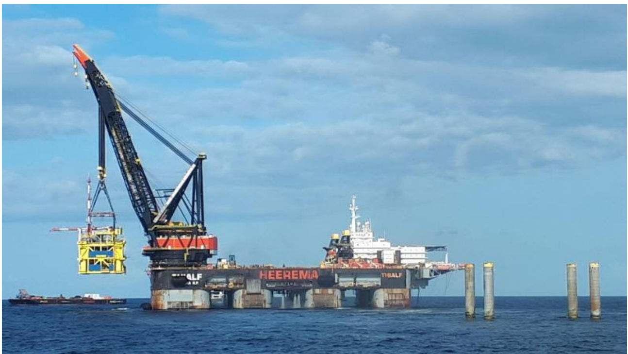
Figure 3.2.2: F3-FA SIP topsides & legs removed separately (photo credit Ocean Energy Resources)
