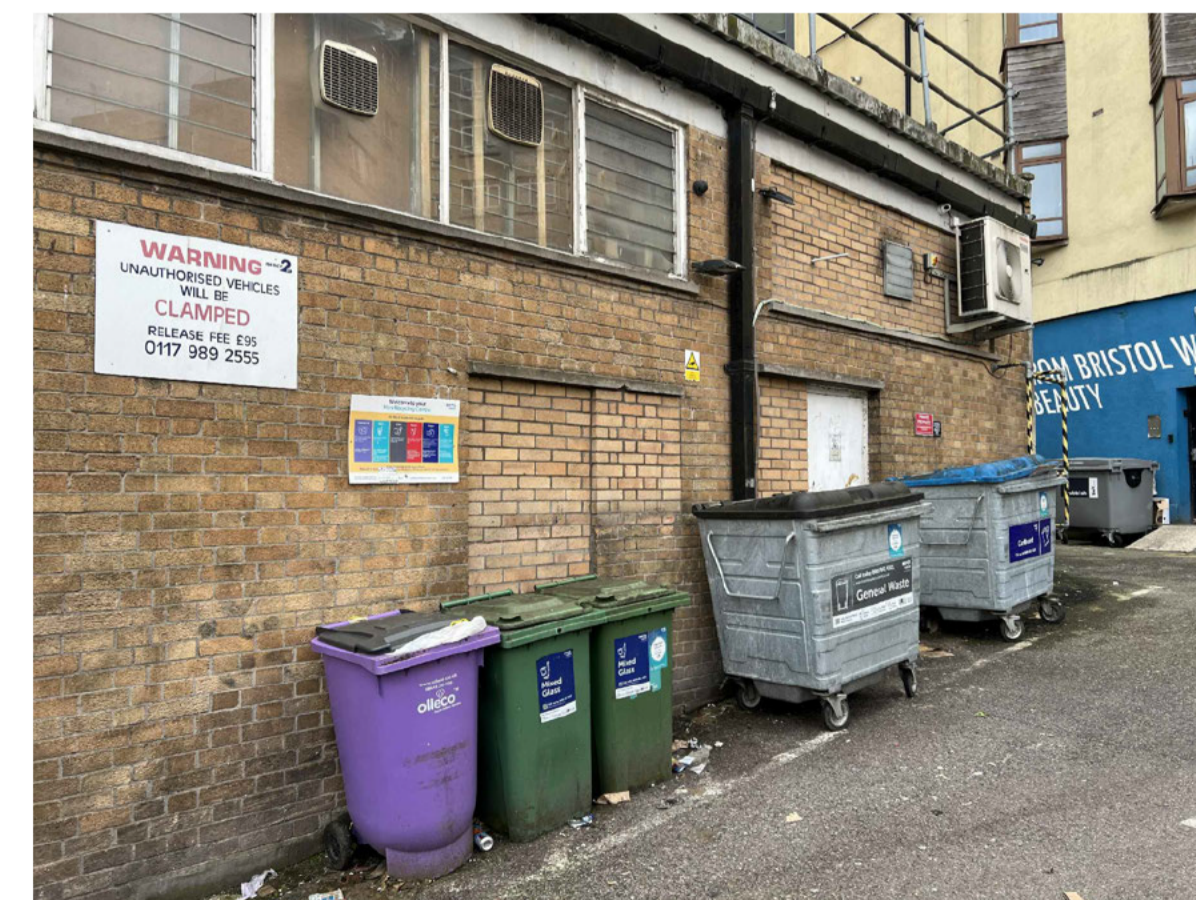
Existing view of North Elevation
