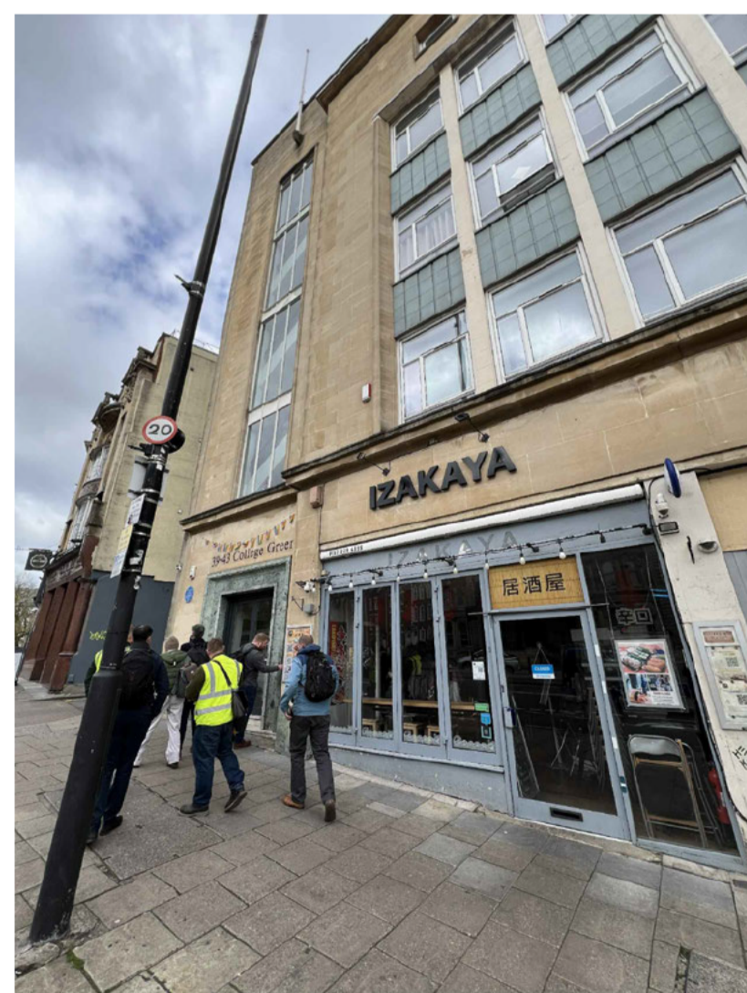
Existing view of South Elevation
