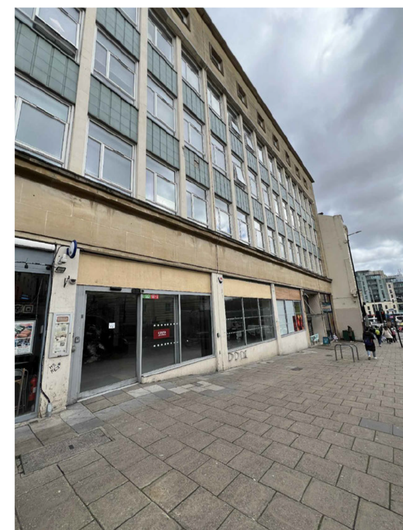
Existing view of South Elevation
