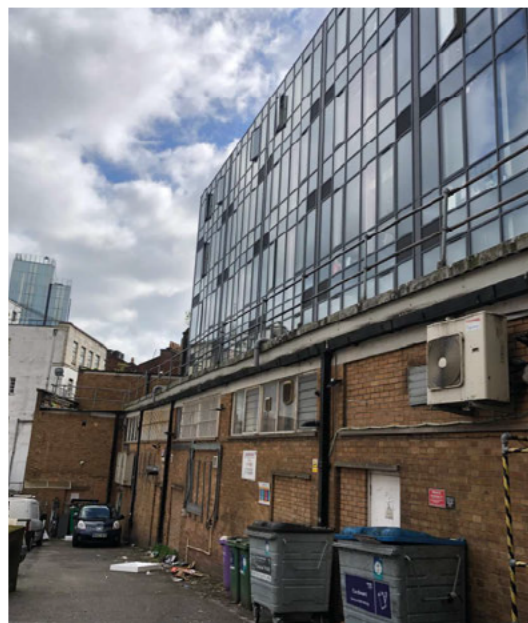
PHOTO 02 - REAR YARD ELEVATION
