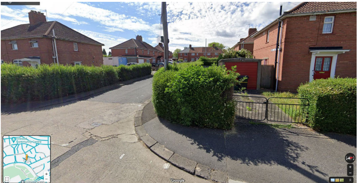
Entrance to Hurst Walk – garages breaking building line
