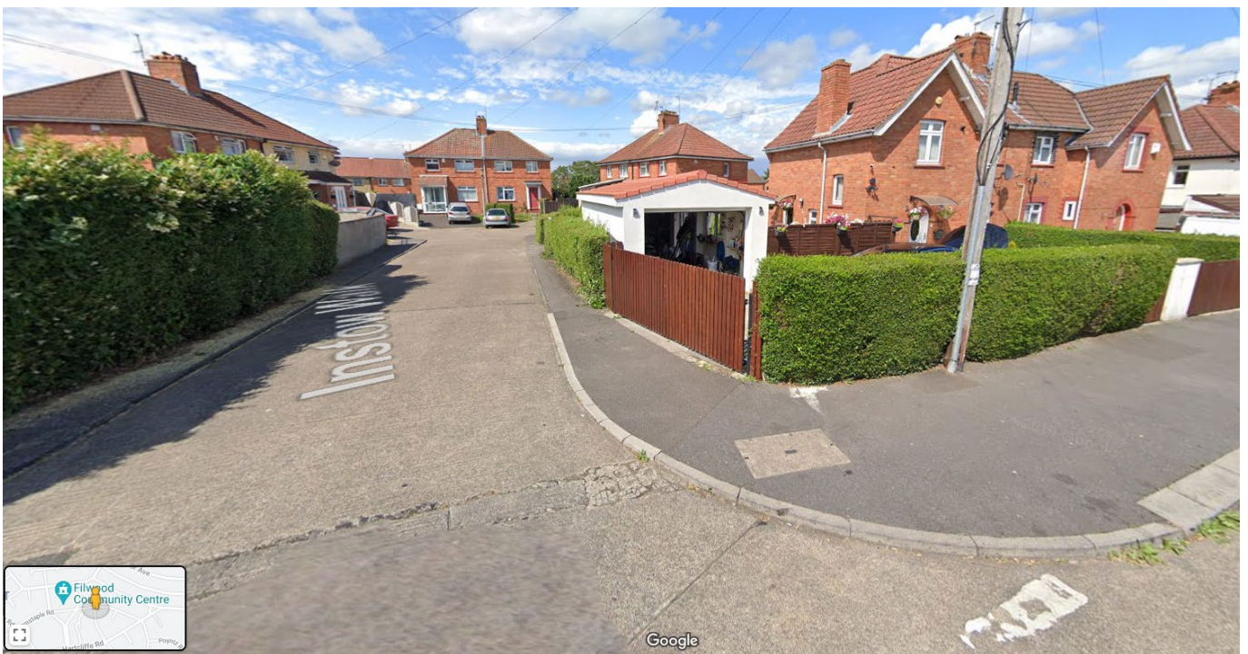
Entrance to Instow Walk – garage breaking building line
