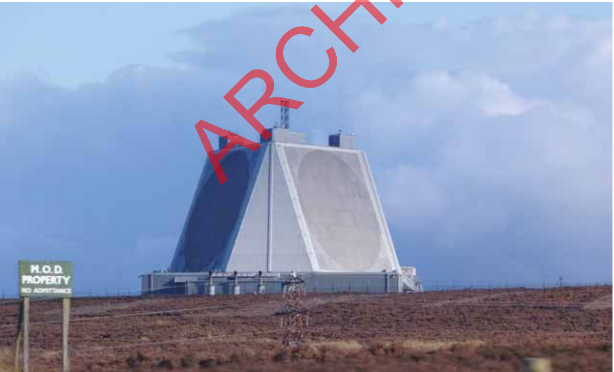
The solid state phased array radar at RAF Fylingdales contributes to UK and United States ballistic missile warning capability
