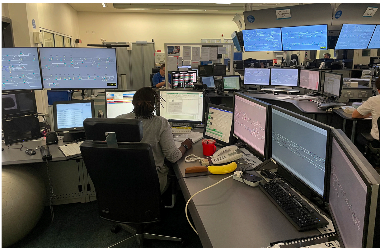
Figure 6: Control room floor at Highgate SCC. Foreground shows desk for line information specialist (LIS) and background shows service controller and other signaller desks.
