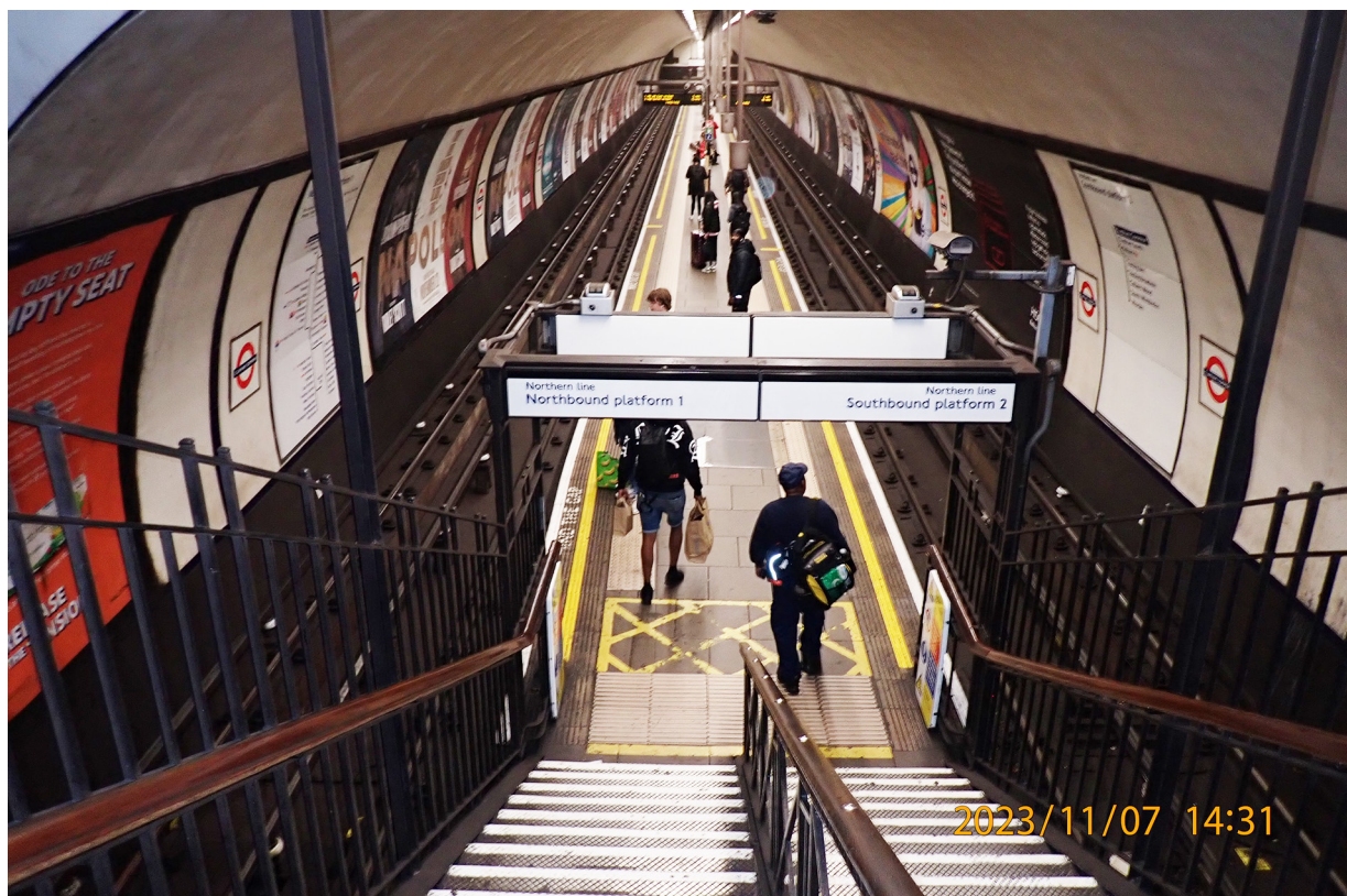
Figure 4: Clapham Common station's island platform from the top of the stairs leading to the platform (northbound line left-hand side and southbound line right-hand side of platform).
