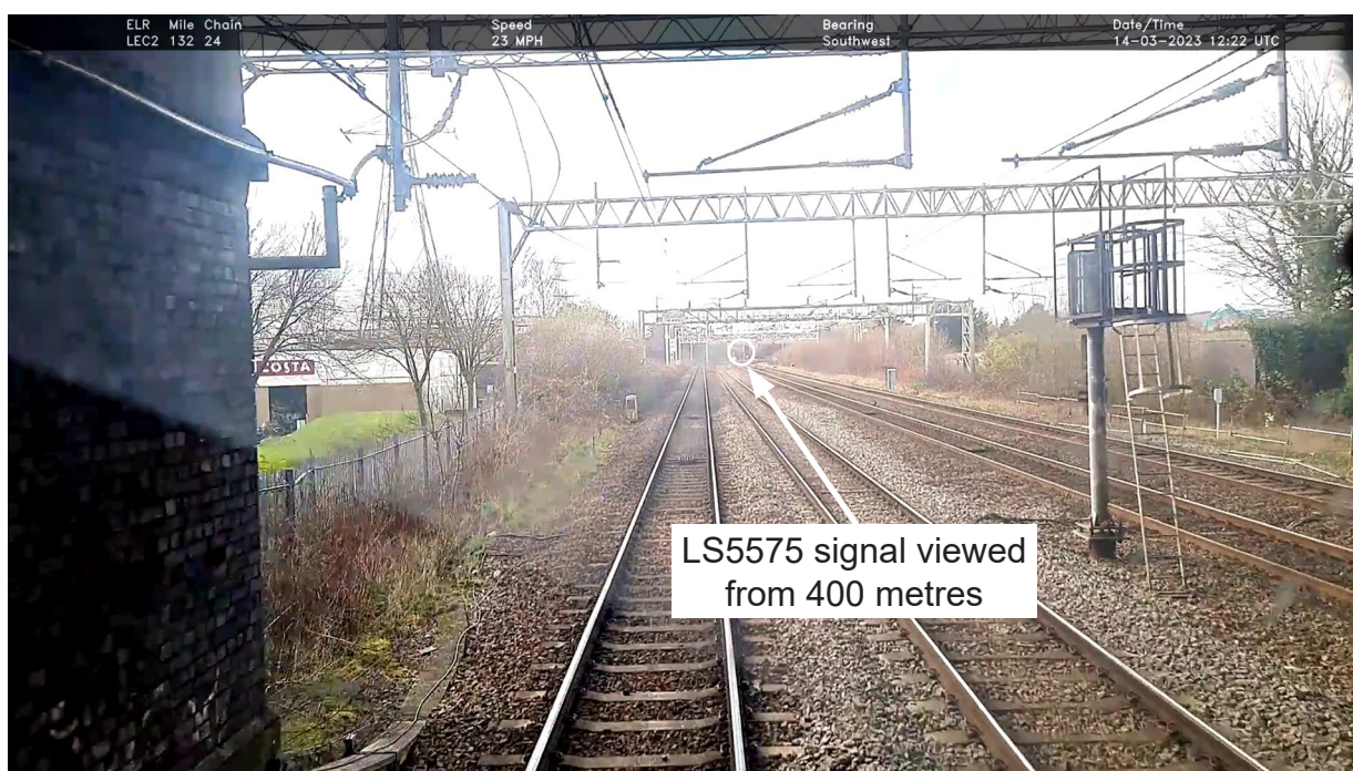
Figure 10: Visibility of signal LS5575 signal (not from the day of the incident) (courtesy of Network Rail with RAIB annotations).
