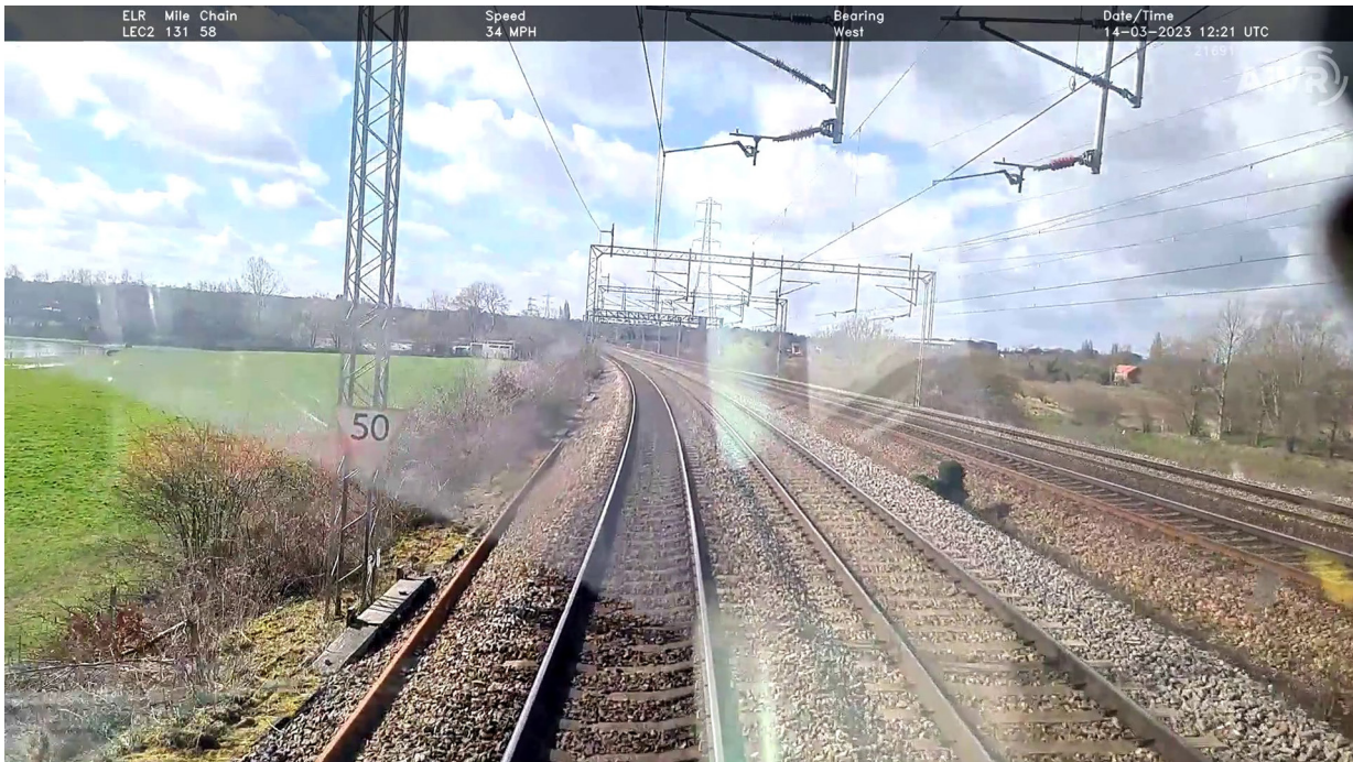
Figure 15: Advance warning sign located on approach to LS5573 signal (courtesy of Network Rail).
