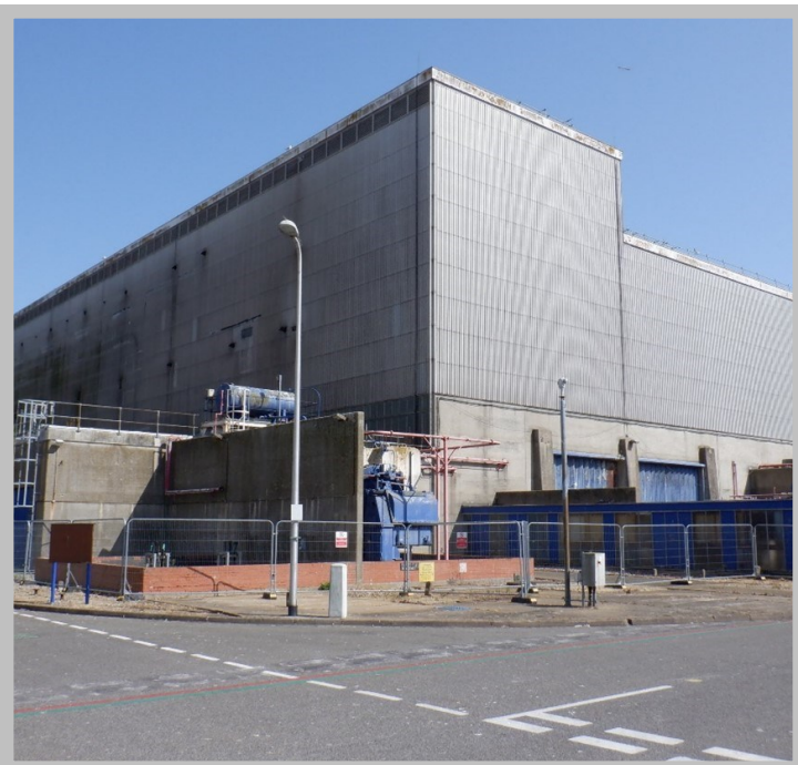
Figure 5: Turbine Hall Building
