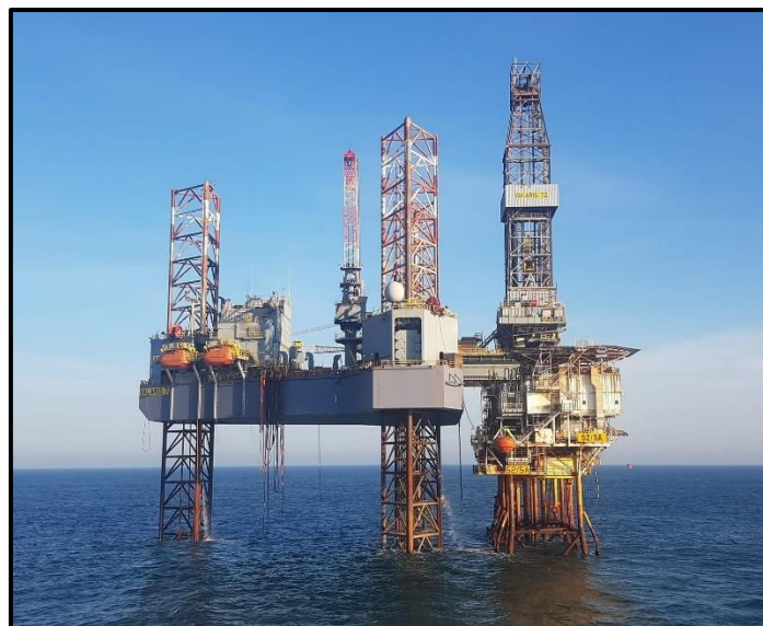
Figure 2: Valaris 72 Jackup alongside 52/5-A Platform
