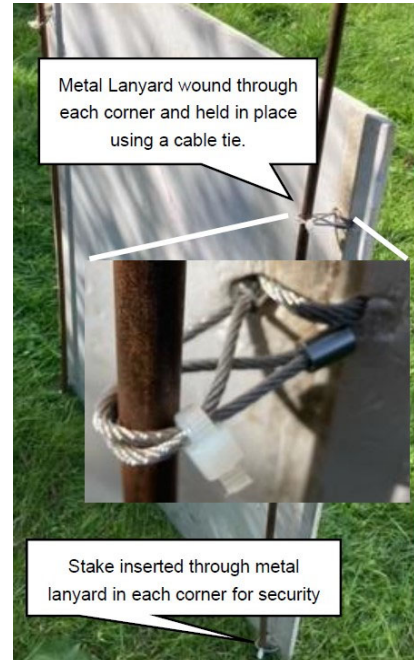
New method of securing the sign (Image used with permission)
