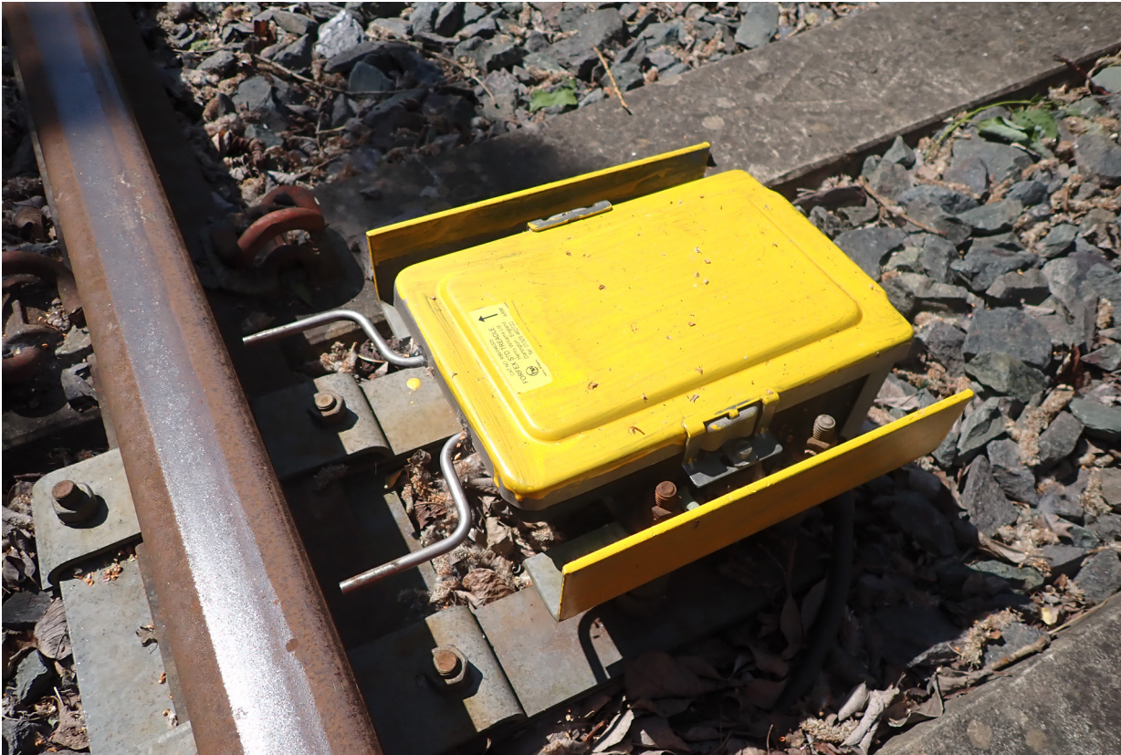
Figure 7: Level crossing 6 strike-in treadle when approached from the exchange sidings.
