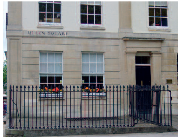
Figure 33: Railings with spear-point finials
