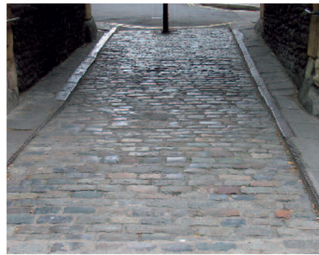
Figure 32: Traditional street surface at St John's on the Wall
