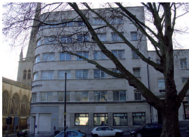
Figure 38: St Nicholas House, High Street
