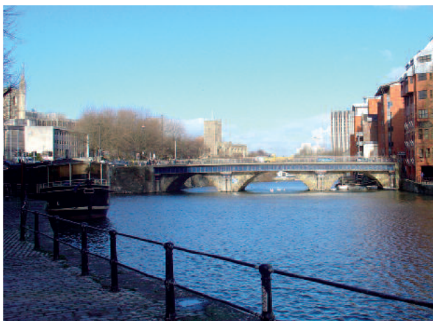
Figure 2: Looking towards Bristol Bridge from Welsh Back
