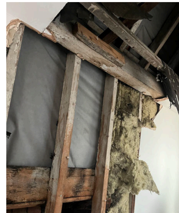
Valley roof construction
