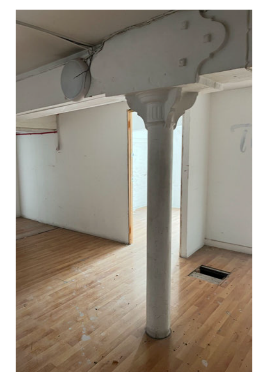
Existing structural columns
