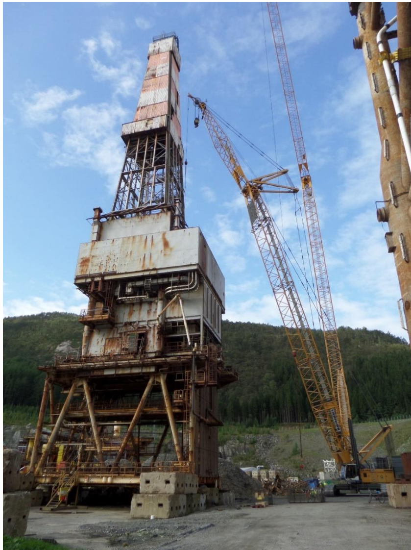
Figure 8-2: On site at Vats
