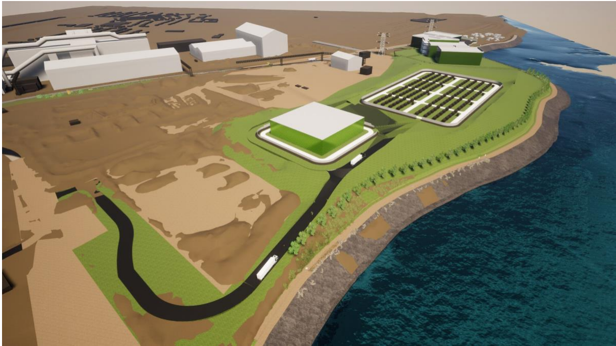
Figure 7: 3D Image of a 1,000 MW Converter Station for a Site in Cardiff
