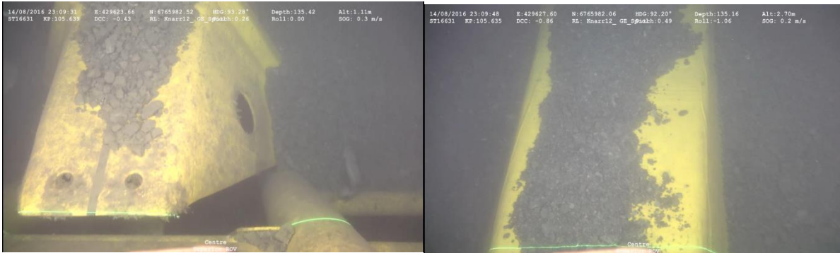
Figure 15 GRP covers close to the PLEM
