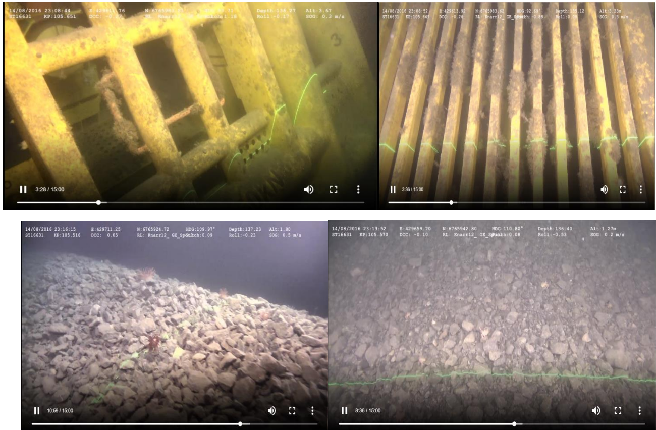
Figure 23 Limited marine growth on the PLEM structure and associated rock cover.
