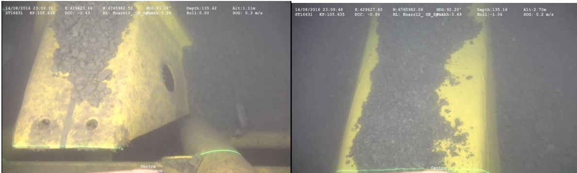
Figure 15 GRP covers close to the PLEM
