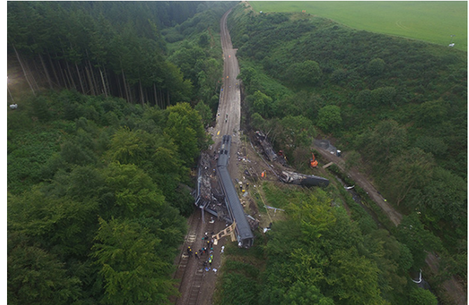
The scene following the accident at Carmont.
