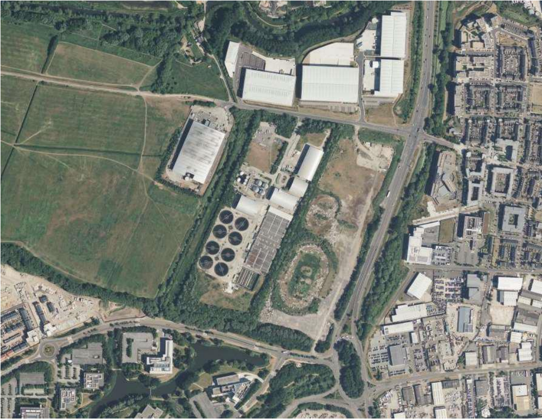
Figure ii Satellite view of Reading Sewage Treatment Works
