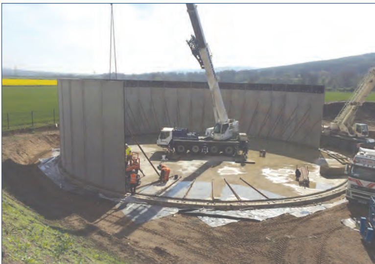
Figure 9.4 A precast concrete segmental tank construction (vertically multi-straked tank) (courtesy A-Consult Ltd)
