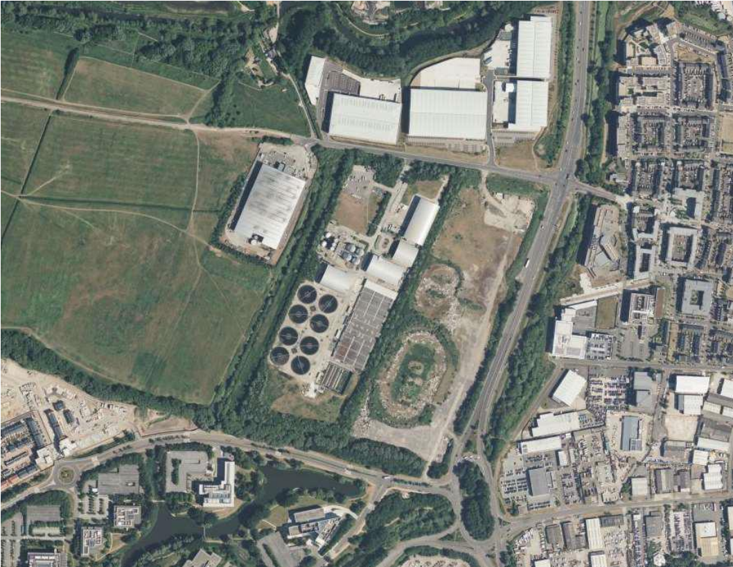
Figure ii Satellite view of Reading Sewage Treatment Works
