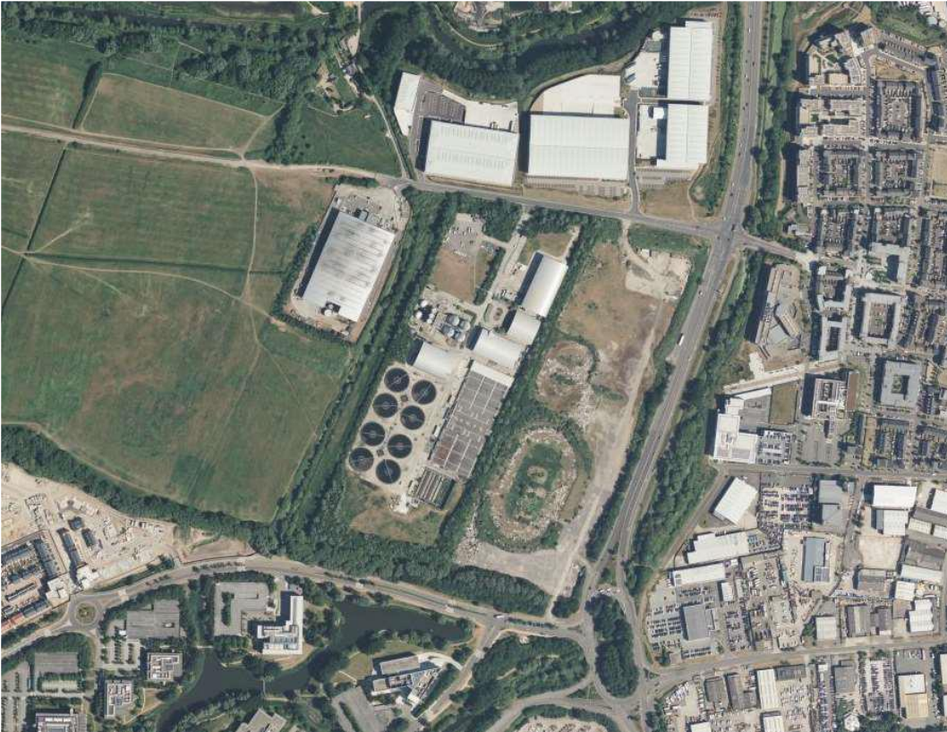
Figure ii Satellite view of Reading Sewage Treatment Works
