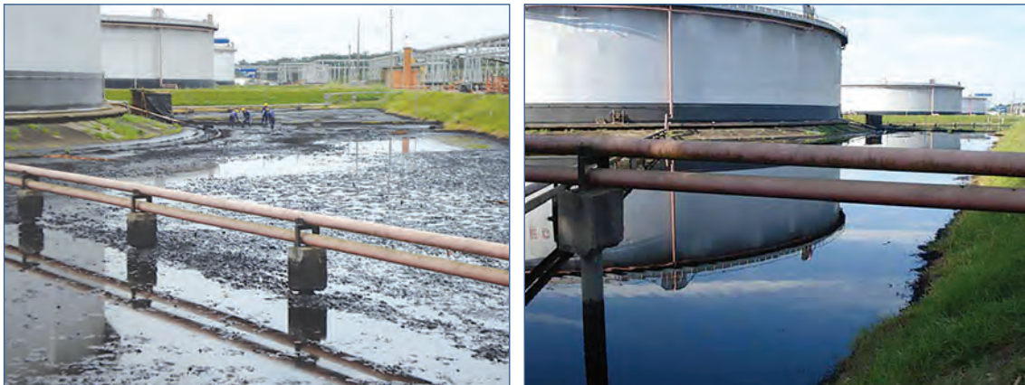
Figure 8.1 Large earth embankment bund (in service) (courtesy Oil Spill Solutions Ltd)
