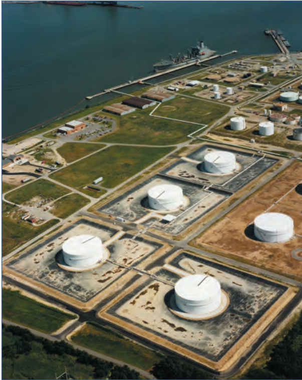
Figure 6.3 A compartmentalised bund (courtesy Seaman Corporation)
