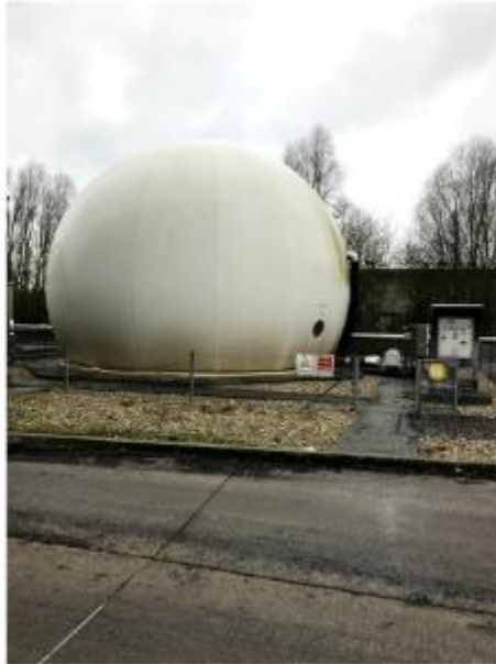
Photo of the one of the site gas holders.
