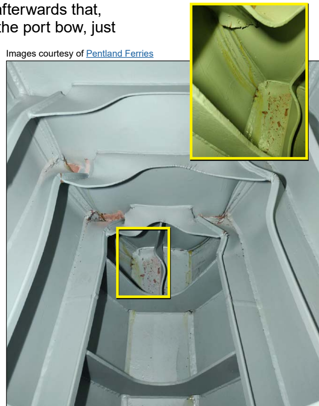
Figure 4: Post-grounding hull damage, showing slight water ingress behind the collision bulkhead
