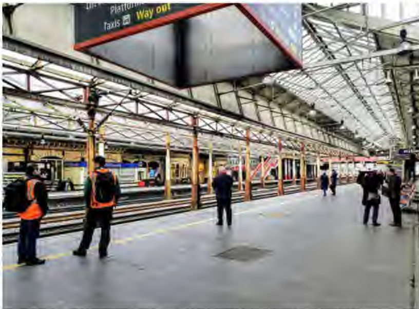
Crewe Railway Station today, HS2 plan to modernise it. (Picture credit: Ryan Parker)
