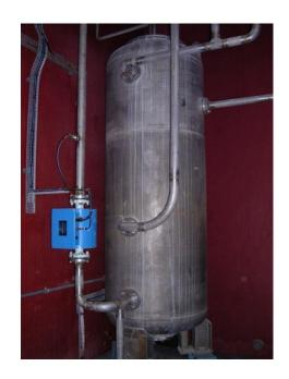
Photograph 6: One of three Caesium Removal Units in the PFP building
