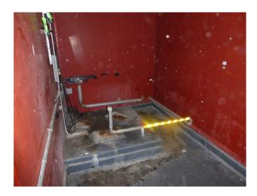
Photograph 8: A Caesium Removal Unit de-planted from one of the three CRU Cells from within the PFP building
