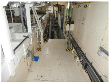
Photograph 3: Floor plates that cover the pond's trench
