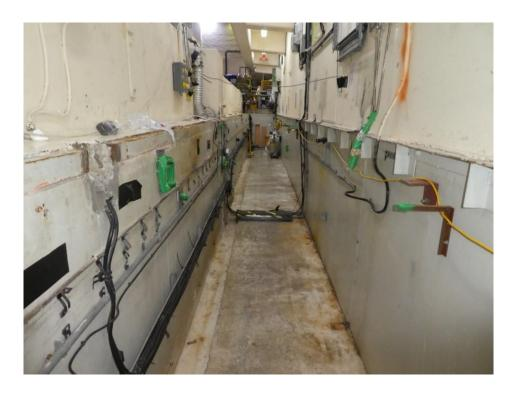
Photograph 5: Pond's trench de-planted of contaminated pipework and ductwork
