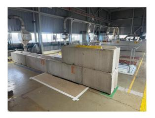
Photograph 31: Construction of the Shield Wall to Protect Operators from Dose
