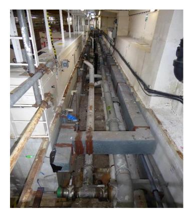
Photograph 4: Contaminated pipework and ductwork within the Pond's trench
