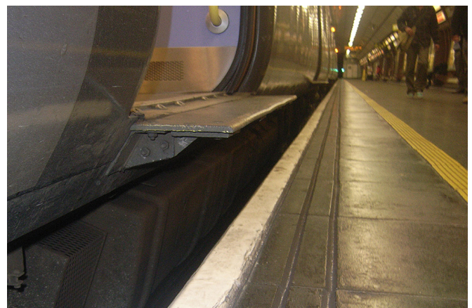
Train doors, step, gap and platform - a hazardous area.
