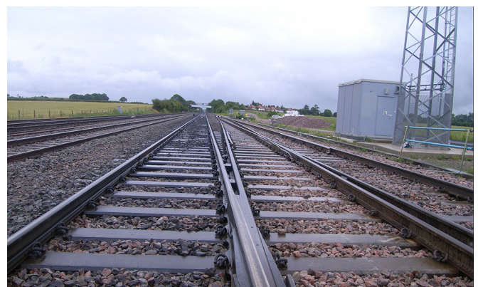
The site of the fatal accident at Ruscombe Junction.
