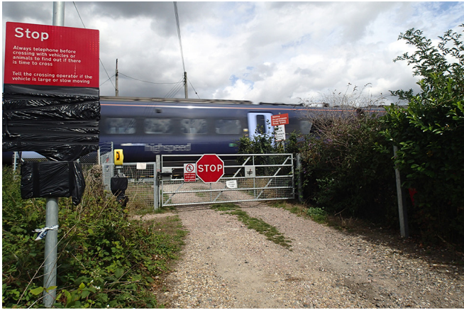
Frognal Farm crossing, after removal of the POGO system following the accident in 2017.
