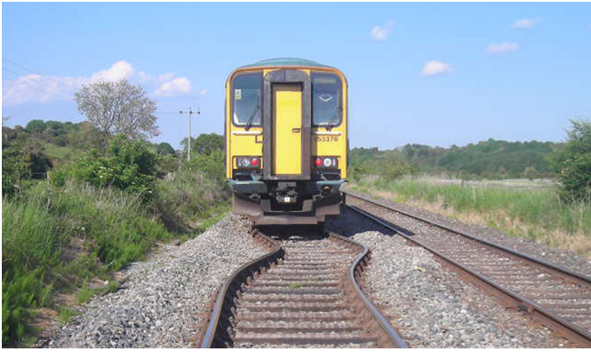
Severe track buckle at Cummersdale.
