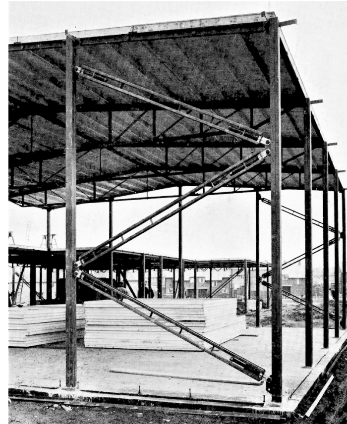
Figure 3: Example of a post-war system build (CLASP)
