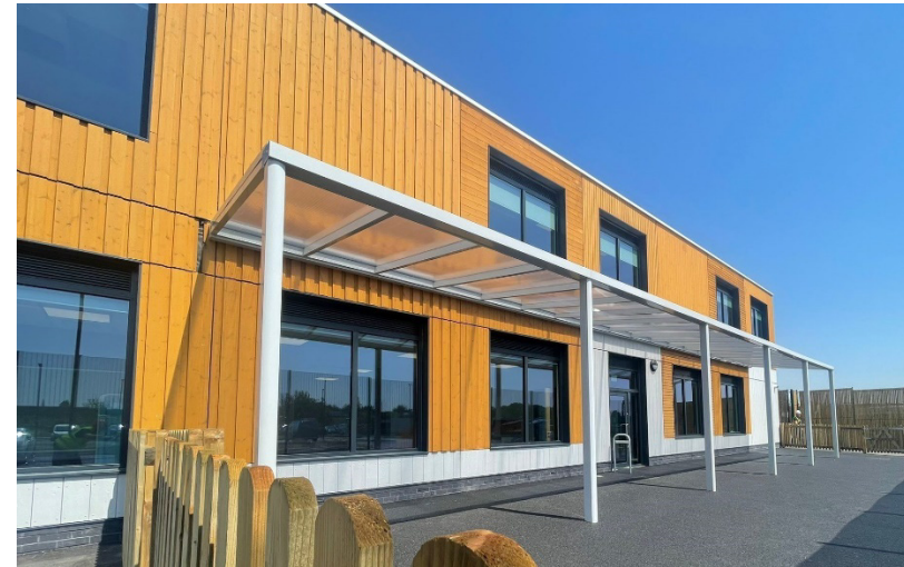
Figure 6: Example of a completed school using MMC/DfMA
