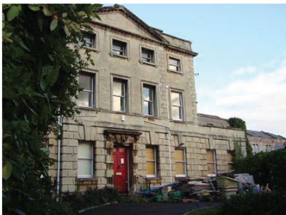
Figure 36: Mortimer House, Clifton Down Road
