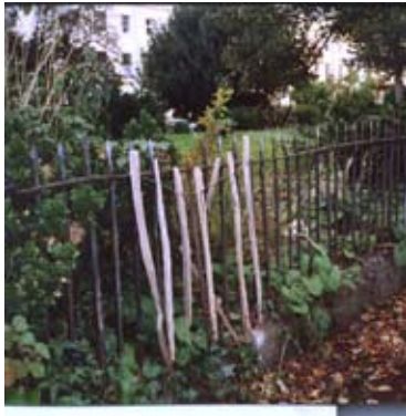
Figure 129: Wooden fence used to plug gap in the railings to a community garden
