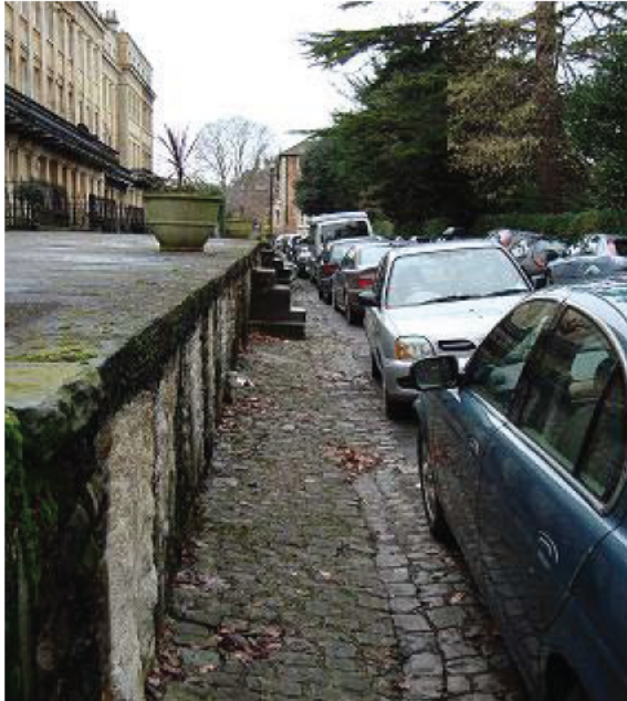
Figure 35: Worcester Terrace raised pavement
