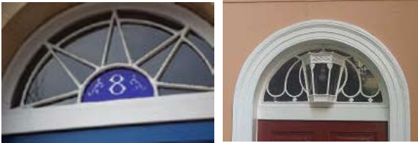
Figure 71: & 72 Wrought iron 'star' fanlight, West Mall; delicate 'Bats wing' fanlight with lantern
