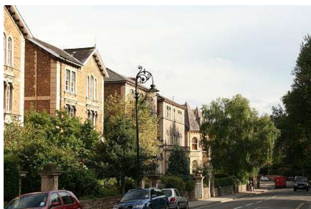
Figure 20: Pembroke Road. These substantial Italianate villas are set in generous landscaped gardens and largely retain much of their original character and appearance. These massive blocks of limestone rubble march confidently up the slope to meet The Downs above. Many have finely detailed Bathstone quoins and window surrounds
