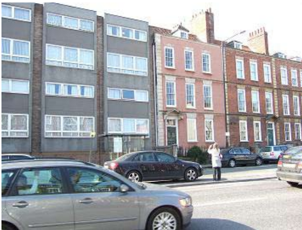
Figure 125: Dowry Parade, the material and fenestration pattern fails to respect that of the Grade II listed properties it adjoins and detracts from the quality of the group and the wider area
