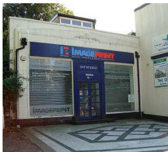
Figure 116: Early 20 th century Art Deco surround with mosaic forecourt, Queens Road
