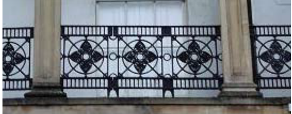
Figure 75: Balcony railing between pilasters, Buckingham Place
