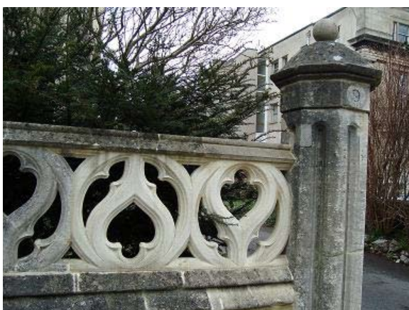
Figure 102: This stone balustrade on Clifton Park has been expertly repaired
