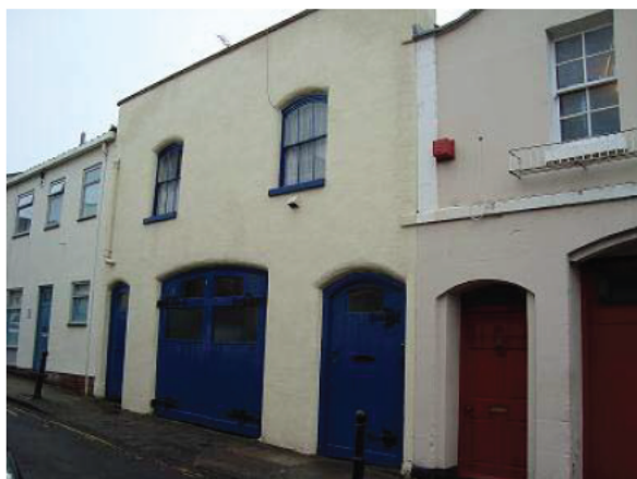
Figure 54: Princess Victoria Street Mews
