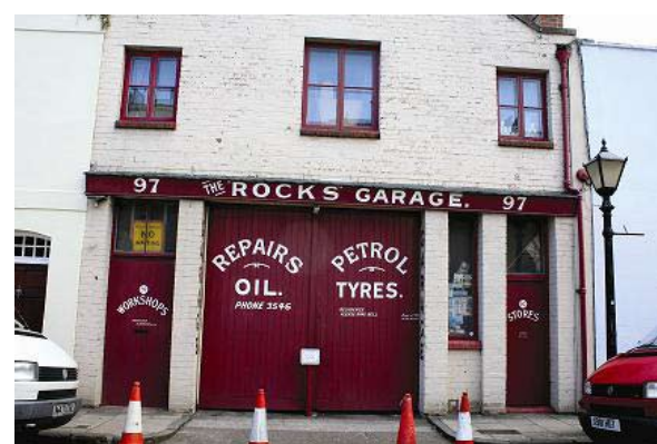
Figure 118: Characterful mews type building, no. 97 Princess Victoria Street
