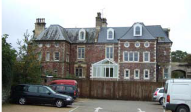
Figure 141: Unauthorised conservatory and dormer window to the rear of Grade II listed Sutton House, Clifton Down. Removed after a court case
