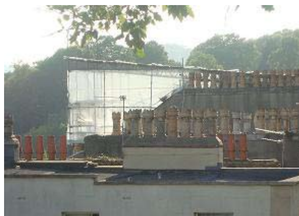
Figure 61: Chimney stacks and pots along the skyline
