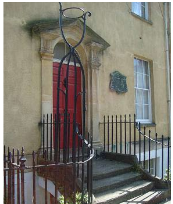
Figure 103: Original oil light fitting attached to wrought iron area railings
