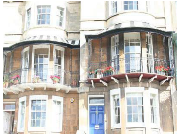
Figure 77: Bowed canopies, Sion Hill
