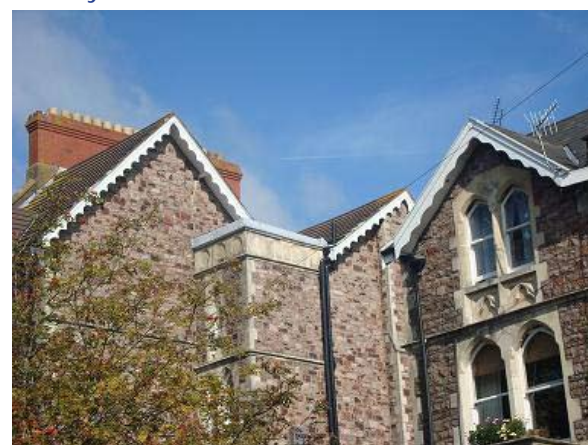
Figure 62: A variety of white painted barge boards appear on later Victorian buildings
