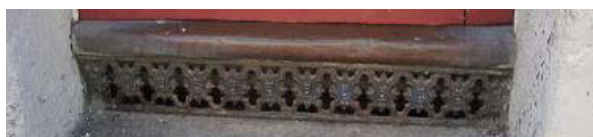
Figure 86: Decorative brass door vent, Ambra Vale
