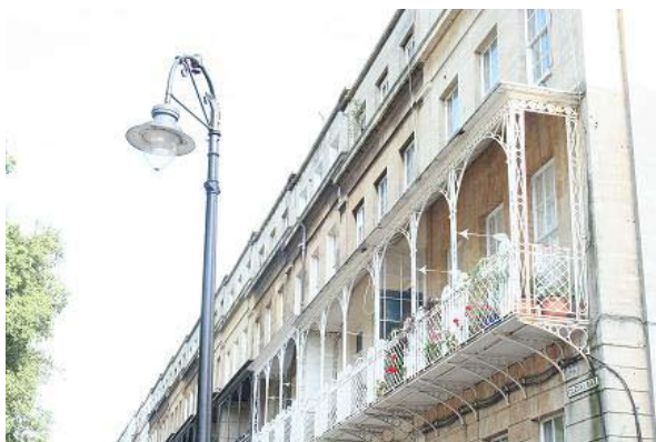
Figure 52: Balconies nos. 1-2 Caledonia Place
