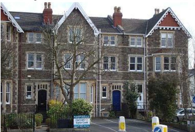
Figure 121: The garden on the right has lost the whole of its boundary wall and been surfaced for car parking. This impacts on the street and terrace as well as individual property and causes run-off during heavy rainfall leading to blocked drains and flooded roads
