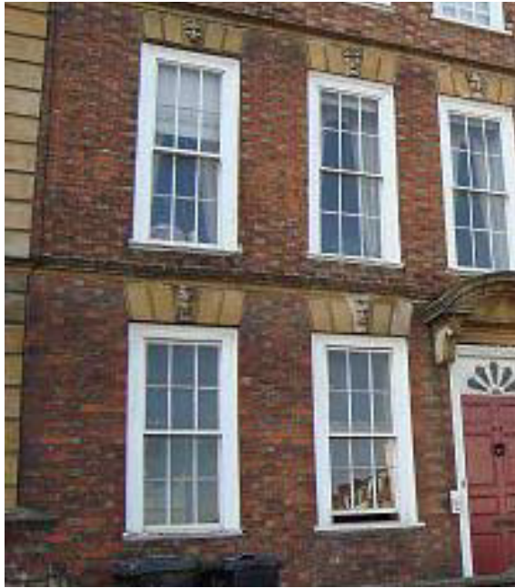
Figure 63: Early 6-over-6 timber sashes, Dowry Parade, flush with the brick facade
