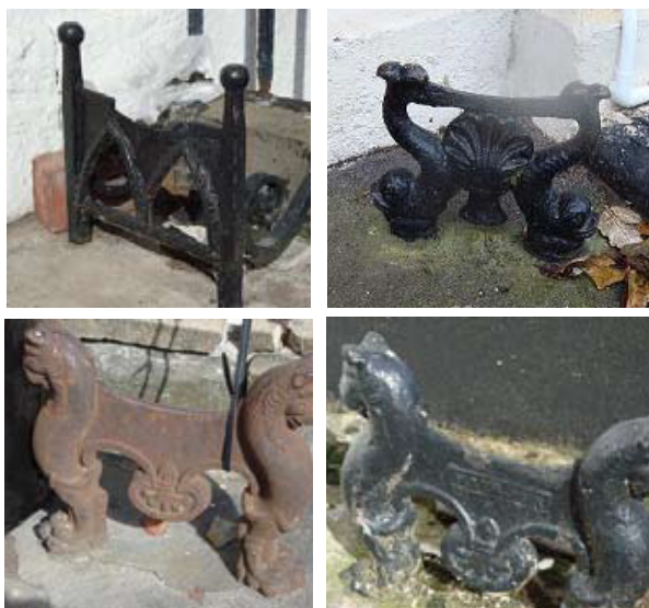
Figure 80-83: Various designs of cast iron footscrapers, many survive in the Clifton Spa terraces
