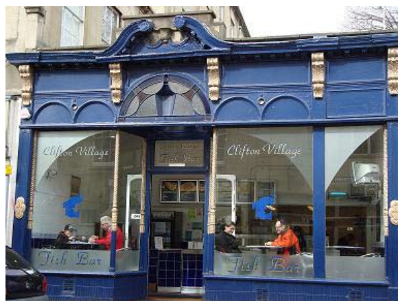
Figure 115: Elaborate timber shopfront, Princess Victoria Street
