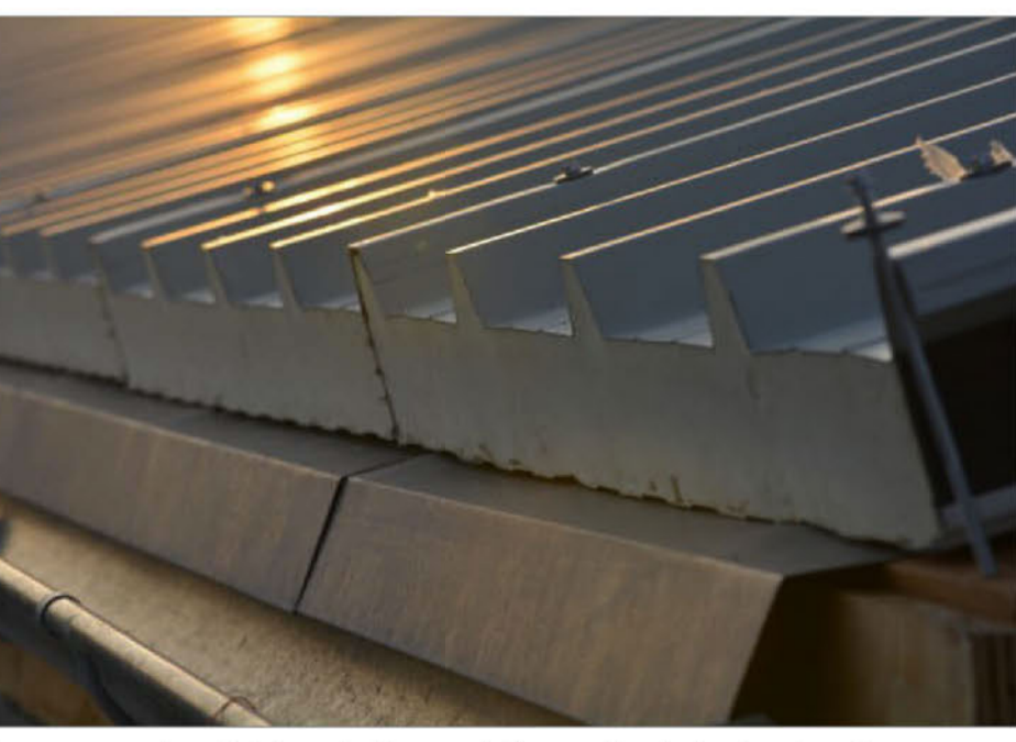
Corrugated Steel Sheet Sandwich to huts
