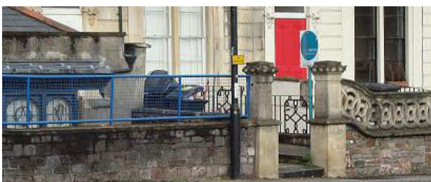
Figure 122: unsympathetic replacements railings detract from the stone balustrade opposite
