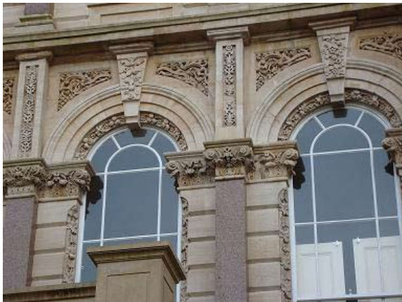
Figure 64: Victorian round-headed sashes with unusual glazing bar pattern
