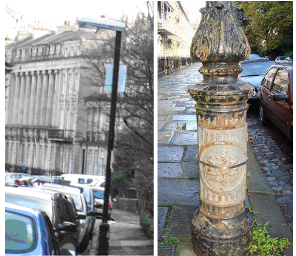
Figure 138-39: An unsympathetic modern replacement lamp standard adjacent to Grade II* Vyvyan Terrace and Christchurch; Grade II lamp standard in poor state of repair
