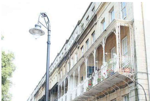
Figure 52: Balconies nos. 1-2 Caledonia Place
