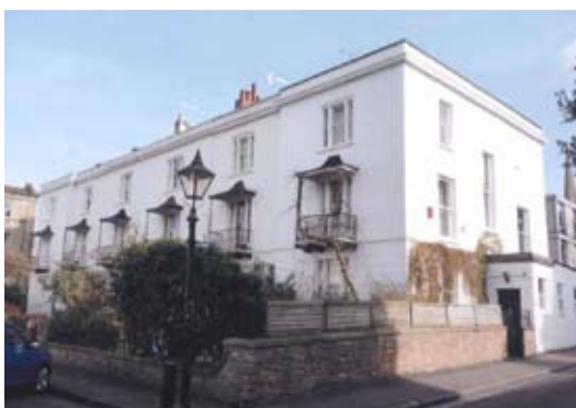
Figure 32: Rear of Canynge Square villas, formerly Somerset Place
