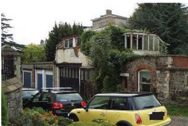
Figure 133: Traditional garage has been left to rot and overgrown with vines. The negative impact is on the character of this mews street which feels neglected and on the traditional garages that are worthy of retention and sympathetic restoration
