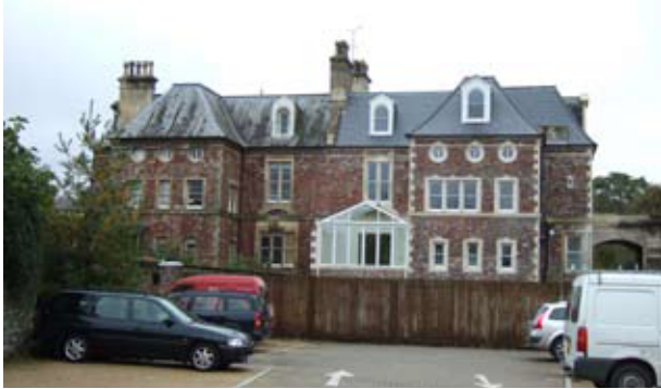
Figure 141: Unauthorised conservatory and dormer window to the rear of Grade II listed Sutton House, Clifton Down. Removed after a court case
