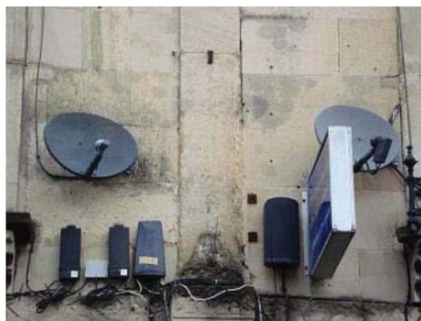
Figure 134: Satellite dishes on the sides of listed buildings are not acceptable. Unauthorised dishes can be enforced against and the owners required to remove them
