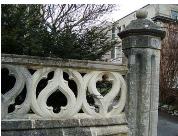
Figure 102: This stone balustrade on Clifton Park has been expertly repaired
