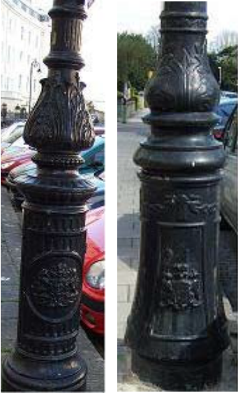
Figure 106-107: There is great variety between cast iron lamp standard bases
