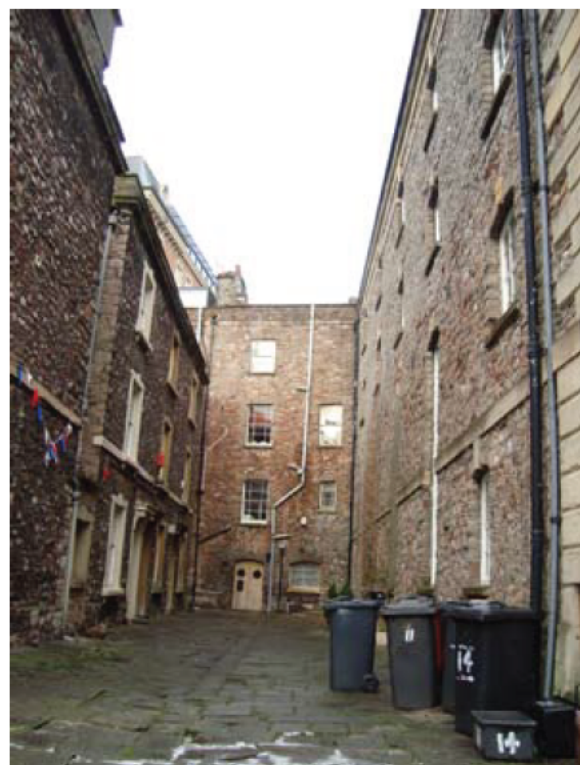
Figure 54a: Carters Buildings, off Portland Street West
