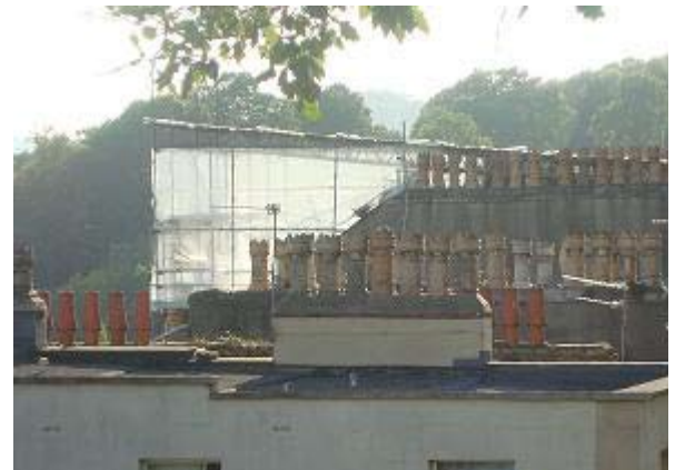
Figure 61: Chimney stacks and pots along the skyline
