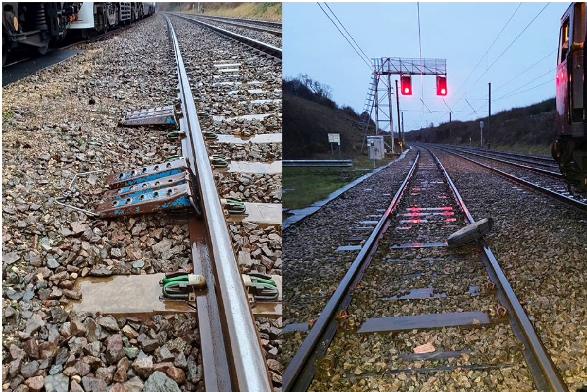
Remains of the portable RRAP found on track. Still in situ metal ramps (left). Displaced foam ramp (right). (Images courtesy of Network Rail.)
