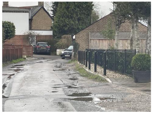
It is proposed to widen the carriageway in the vicinity of The Hollies. There are existing bollards in this location, which are positioned close to the kerbing. There will be insufficient clearance between the new kerb and the bollards. This may result in vehicles colliding with the bollards.
