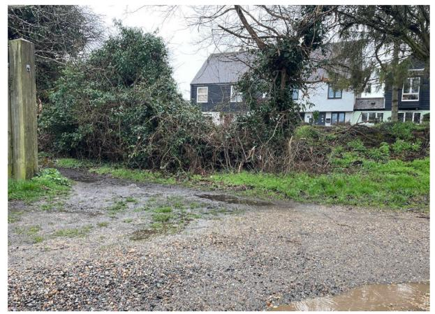
Site observations reveal a significant difference in the levels between Mill Lane and Home Pastures, which may result in a steep gradient on the pedestrian/cycle connection. This may result in users tripping or falling whilst negotiating the path.
