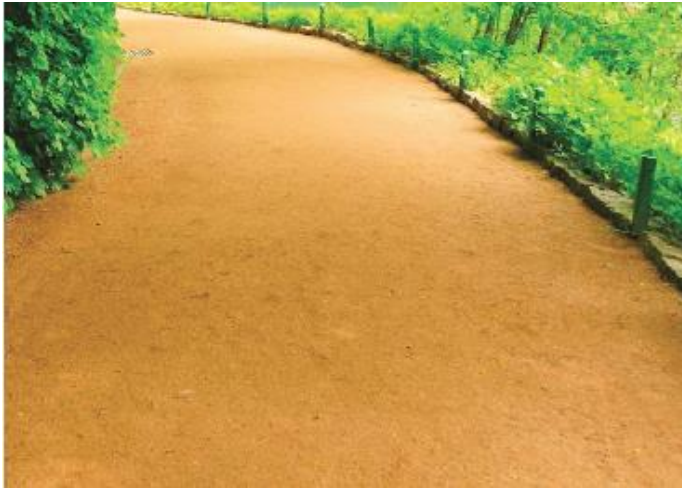
Fig. 8 - Hoggin bound gravel surfacing
