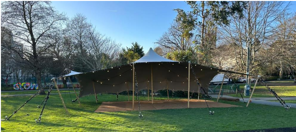
Fig. 4 – Example Tent Structure
