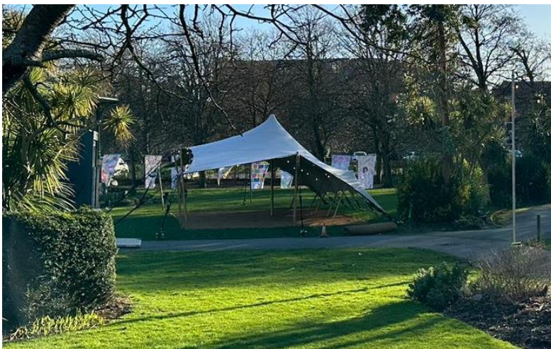
Fig. 5 – Example Tent Structure
