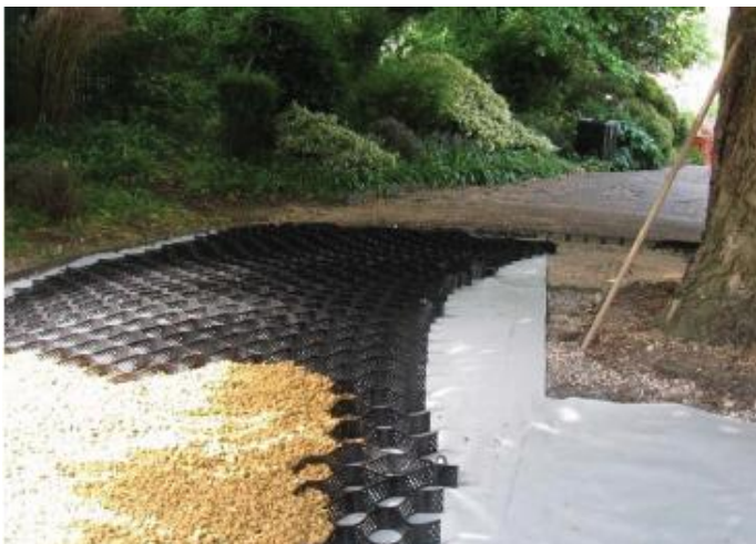
Fig. 10 – Cellular grid systems within existing tree rooting areas
