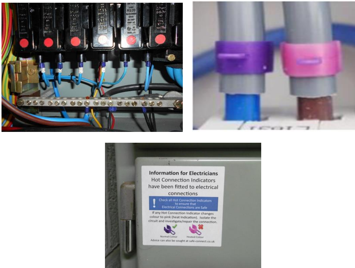
Figure 3.1: Cable hot connection indicators
