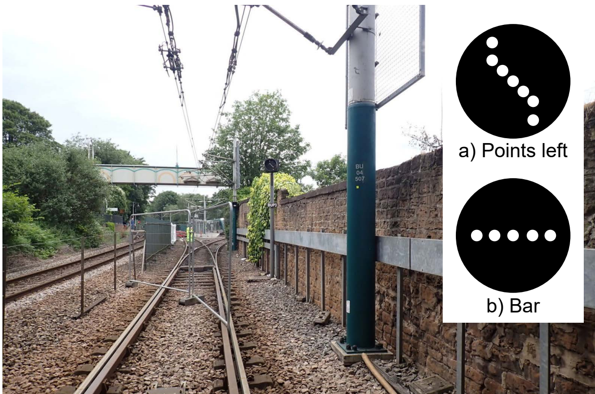
Figure 6: The FPI alongside BUP3 points, and (inset) the two possible indications that the FPI can show to drivers: a) Points left and b) Bar.
