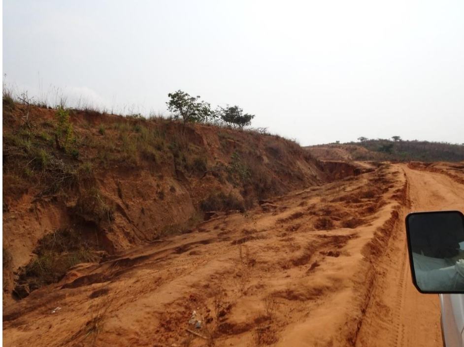
Figure 62 - Unpaved access road to the Municipality of Buengas
