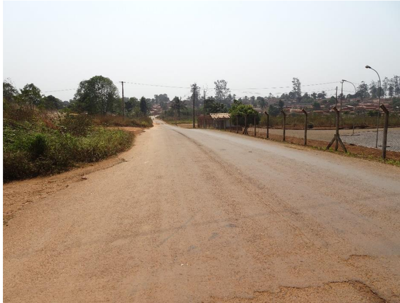
Figure 126 – Access Road to Negage substation
