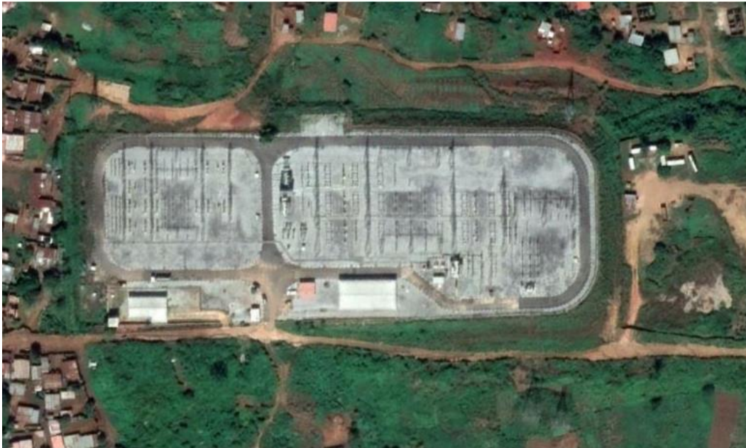
Figure 125 – Surrounding the Uíge substation, next to a residential area
