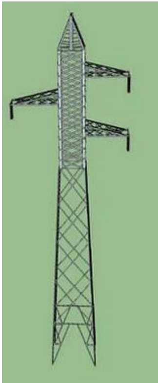
Figure 18 – Example of 110 kV transmission towers
