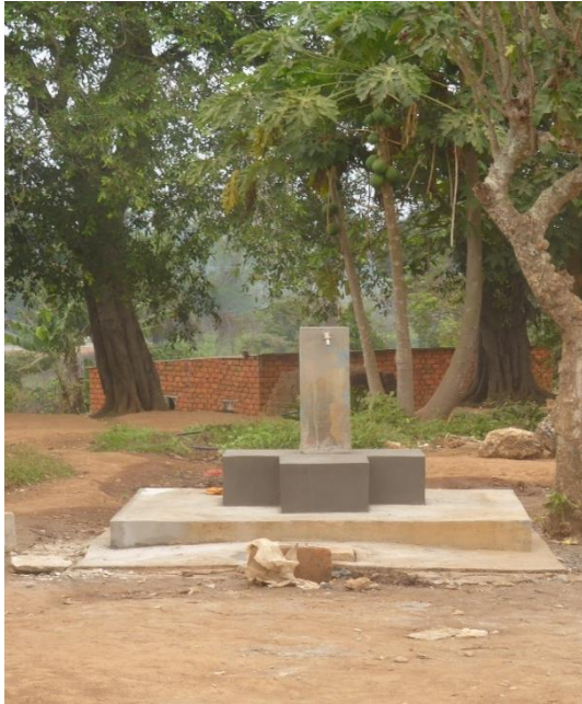
Figure 51 – Borehole in Uíge
