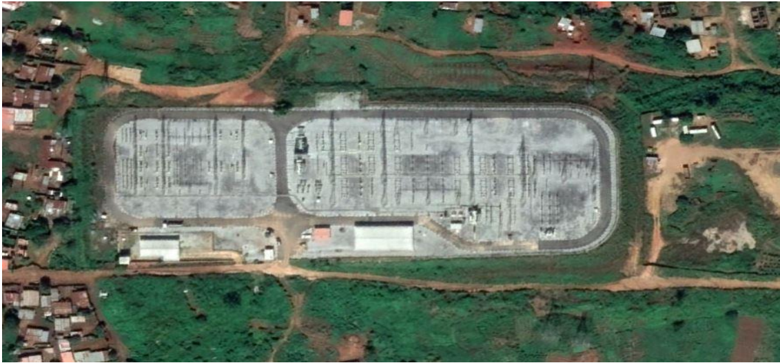
Figure 16 – Current situation of the Uíge Electricity Substation
