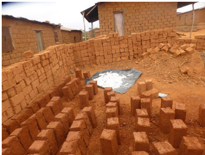
Figure 123 – Adobe brick manufacturing
