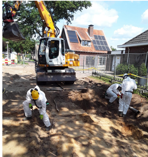
Removing asbestos contaminated soil | NTP
