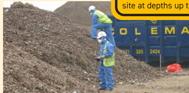
Asbestos finds—hand picking | Ramboll
