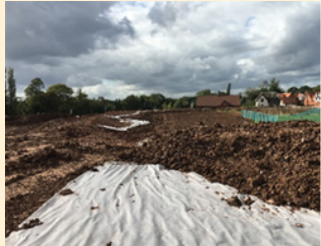
Installation of the cover system | AECOM
