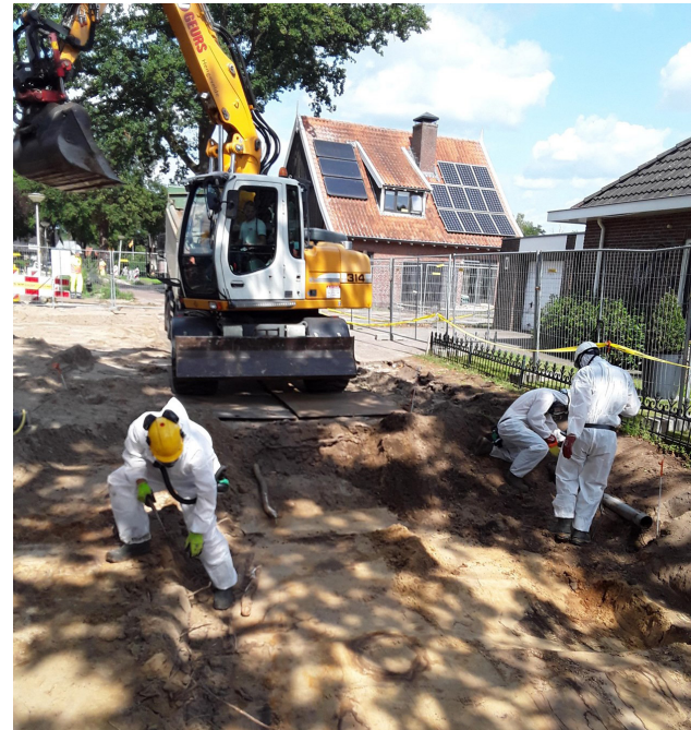
Removing asbestos contaminated soil | NTP
