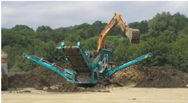
Mechanical screening of excavated soil | AECOM
