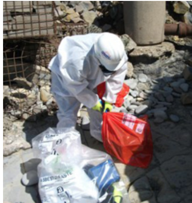
Double bagging of asbestos waste in UK | Ramboll
