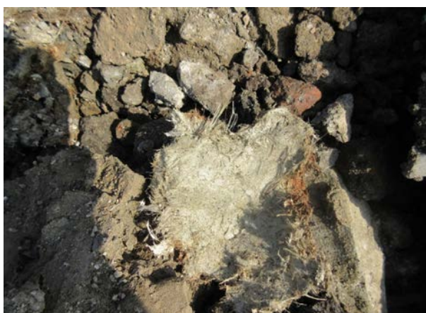
Photo courtesy of Hydrock. Plate 23. Highly degraded/disaggregated AIB/fibrous board in excavated made ground.
