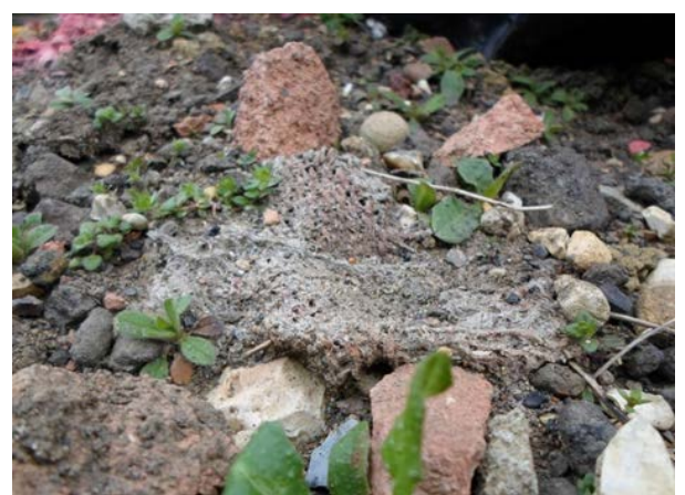
Photo courtesy of Hydrock. Plate 16. Weathered asbestos textile on surface of made ground.
