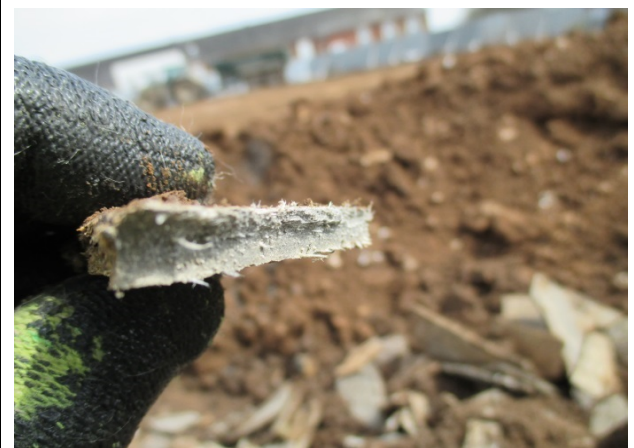
Photo courtesy of VertaseFLI. Plate 6. Close-up shot of degraded asbestos insulating board (AIB) fragment collected from excavation.
