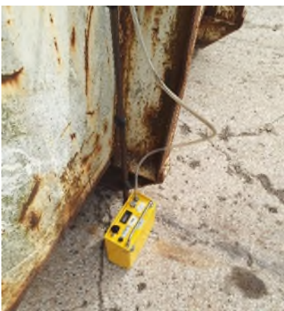
Photograph 30 – 07/09/23 Adjacent SEM Sample point (Downwind)
