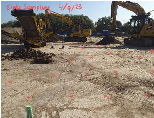
Photograph 9 – 04/09/23 Slab sampling locations
