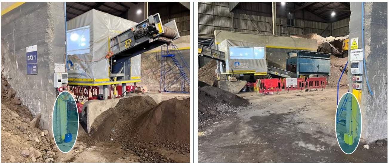
Figure 2.5: Example locations for SEM air monitoring at ERQ
