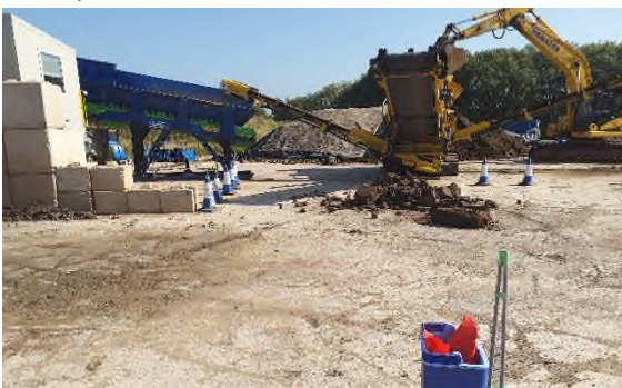
Photograph 5 – 04/09/23 Dust/debris to slab for sampling A
