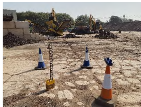
Photograph 23 – 06/09/23 Adjacent SEM Sample point (Downwind)
