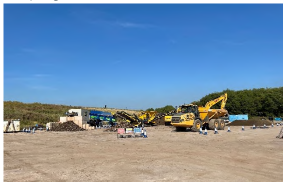
Photograph 8 – 04/09/23 End of the day clean up (@17:55)
