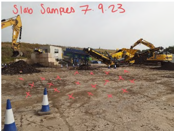
Photograph 32 - 07/09/23 Slab sampling locations
