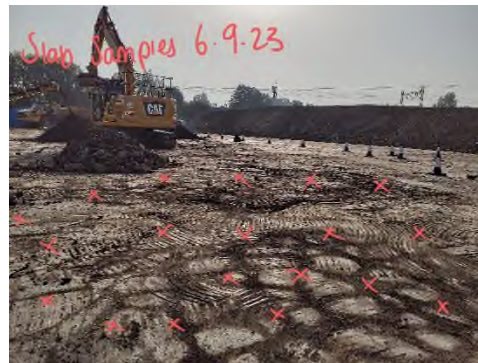
Photograph 25 – 06/09/23 Slab sampling locations
