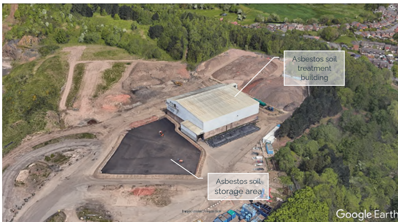
Figure F.16: Google Earth image of STF and asbestos soil treatment building for context
