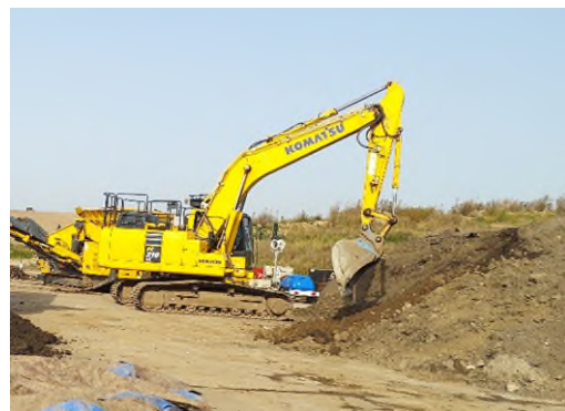
Photograph 20 – 06/09/23 pre-screened material stockpile
