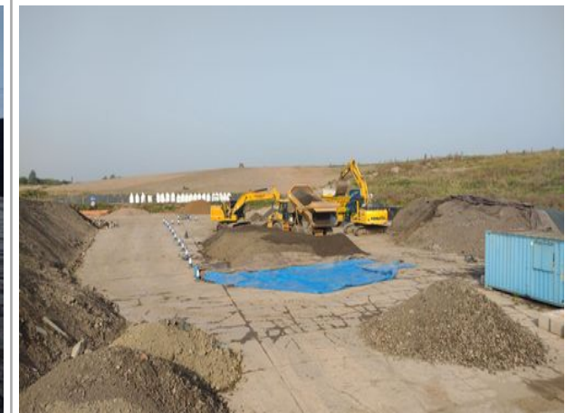
general works area photo
