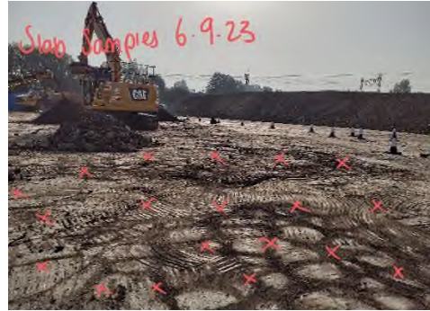
Photograph 25 – 06/09/23 Slab sampling locations
