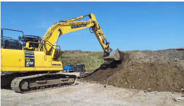
Photograph 3 – 04/09/23 pre-screened material stockpile
