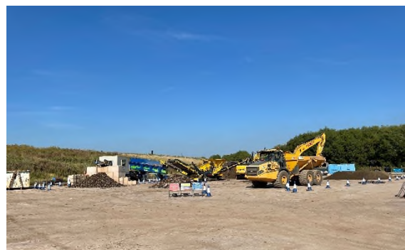
Photograph 8 – 04/09/23 End of the day clean up (@17:55)
