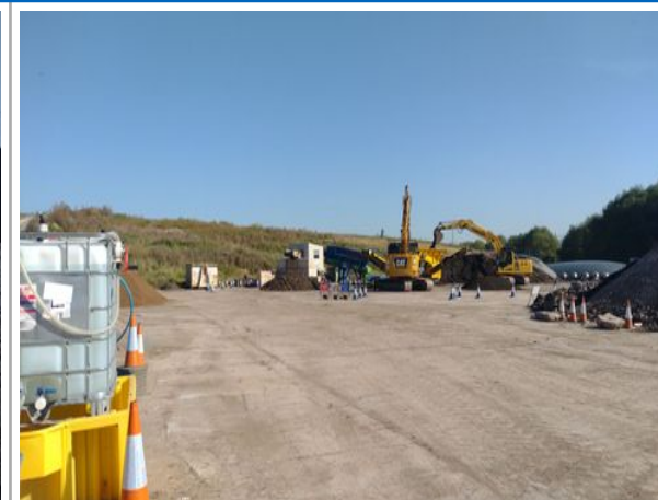
general works area photo
