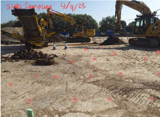
Photograph 9 – 04/09/23 Slab sampling locations
