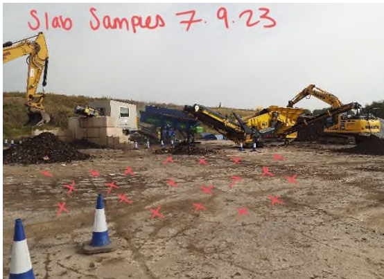
Photograph 32 – 07/09/23 Slab sampling locations
