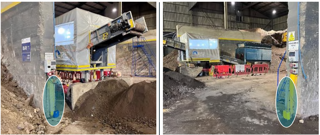
Figure F.20: Example locations for SEM air monitoring at ERQ
