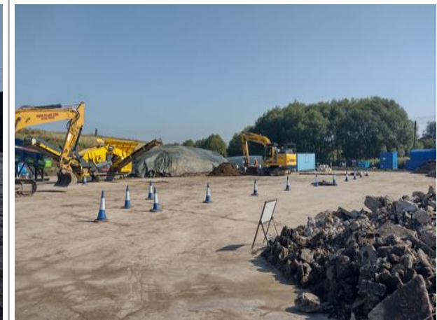
general works area photo
